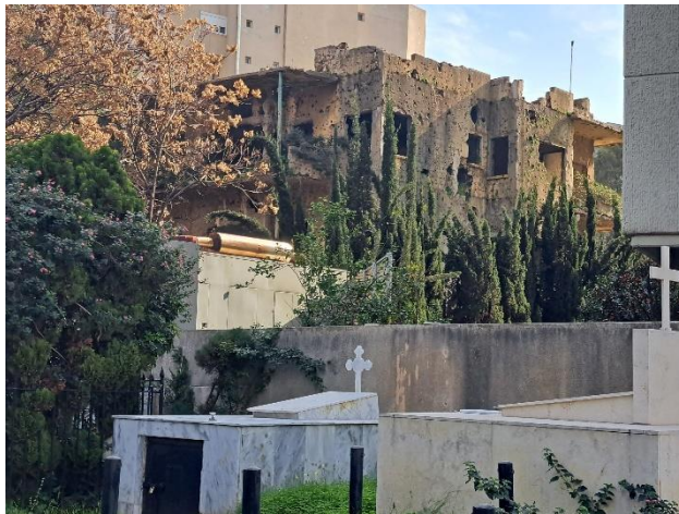
Figure 4. War-damaged building on Beirut's previous demarcation line – Photo Credit: Author N. Hindi – Jan. 2023.
