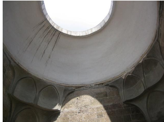
(b) Interior of the dome (by author, 2017)
