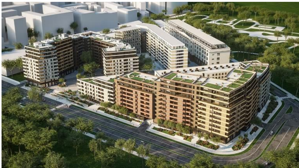
Figure 2. Residential complex "K DISTIRKT" (2022), Belgrade (Source: https://kdistrict.rs/index.html#stanovi/ accessed 21.2.2023.)
