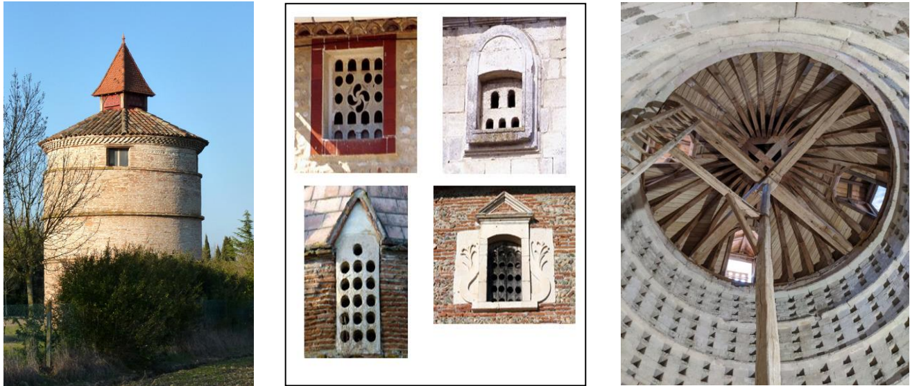
Figure 4. On the left, a circular brick dovecote with a triple randière, topped by a lantern with a flight grille, Château Rouge, Haute-Garonne (France). Source: https://www.alaingillodes.fr/ ; in the center: various examples of flight grilles. Source: https://pigeonniers-et-colombiers-de-france.webador.fr/ ; on the right: a spiral staircase in the Villesavin dovecote, restored in 2019. Source: Wikimedia Commons
