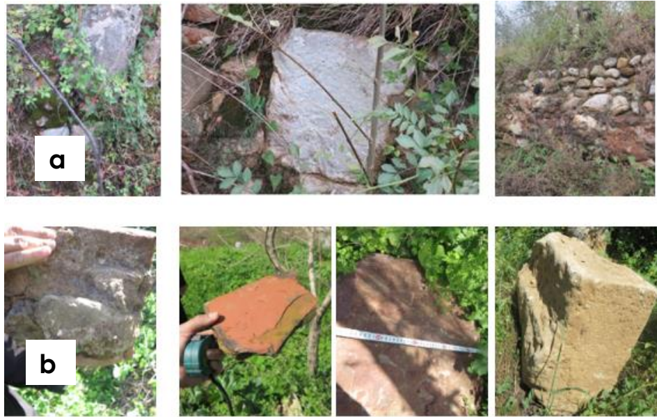
Figure 16. Fragments of retaining walls still standing (a). Wall materials scattered over site 01 (cut stone, bricks, floor tiles) (b).
